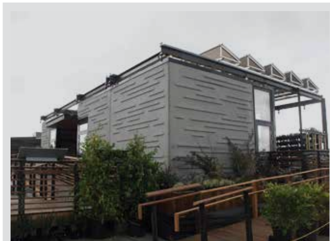
Figure 1. Precast geopolymer cement concrete house.
