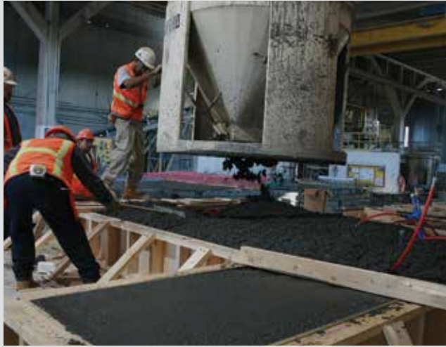
Figure 7. Placing concrete in forms.
