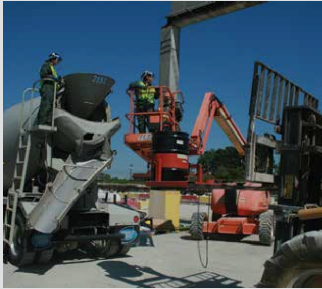
Figure 6. Batching activating solutions into the concrete mixing truck.
